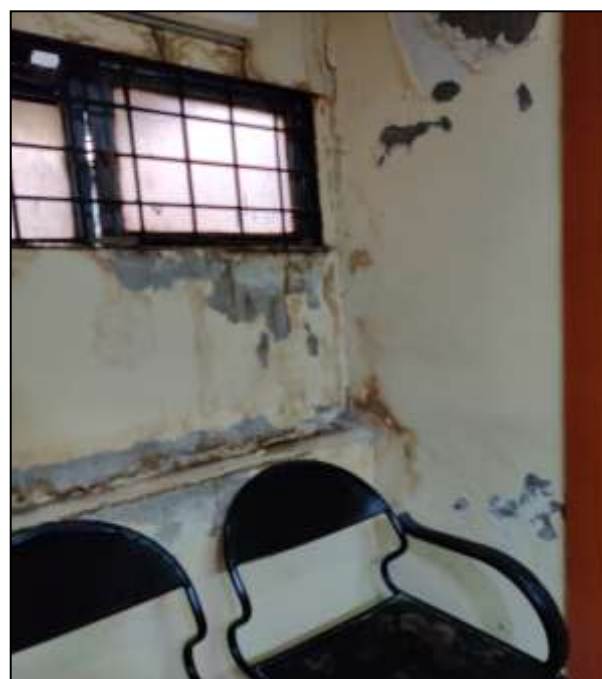
Fig. 10. Leakage and dampness observed in the Bank (lecture room no.4) on the external wall
