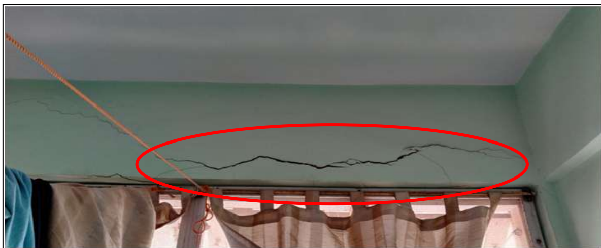
Fig. 28. Horizontal crack in Beam bottom in room no 414
