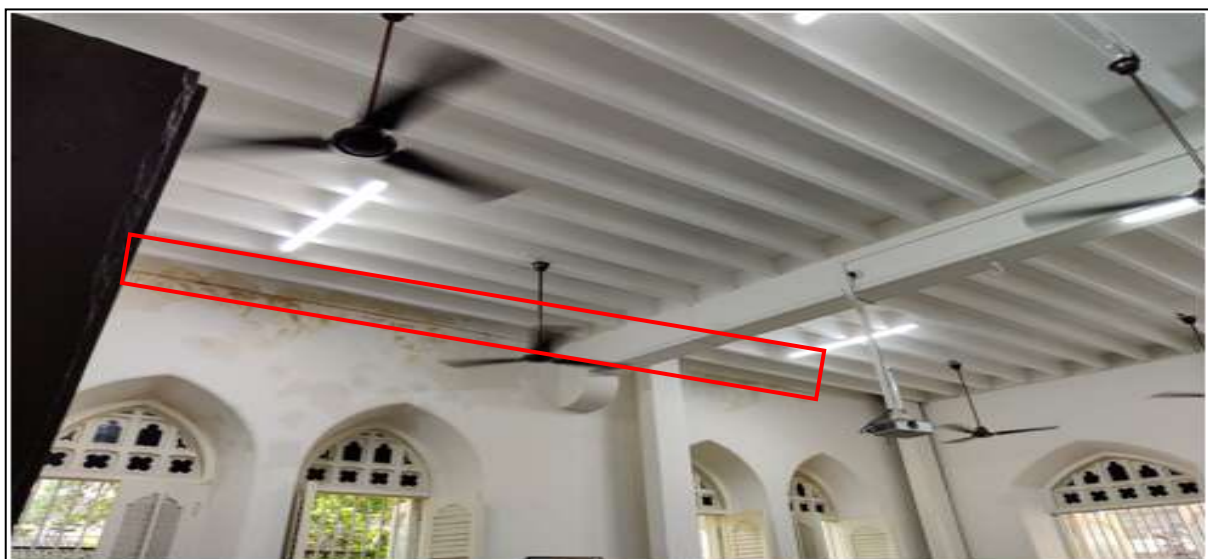
Fig 4. Dampness and leakage marks on first floor office building
