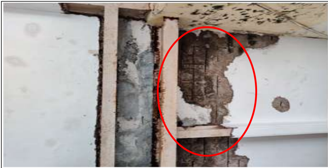
Fig 14. Exposed reinforcement in landing area of stair case between Hall Building and Science Building
