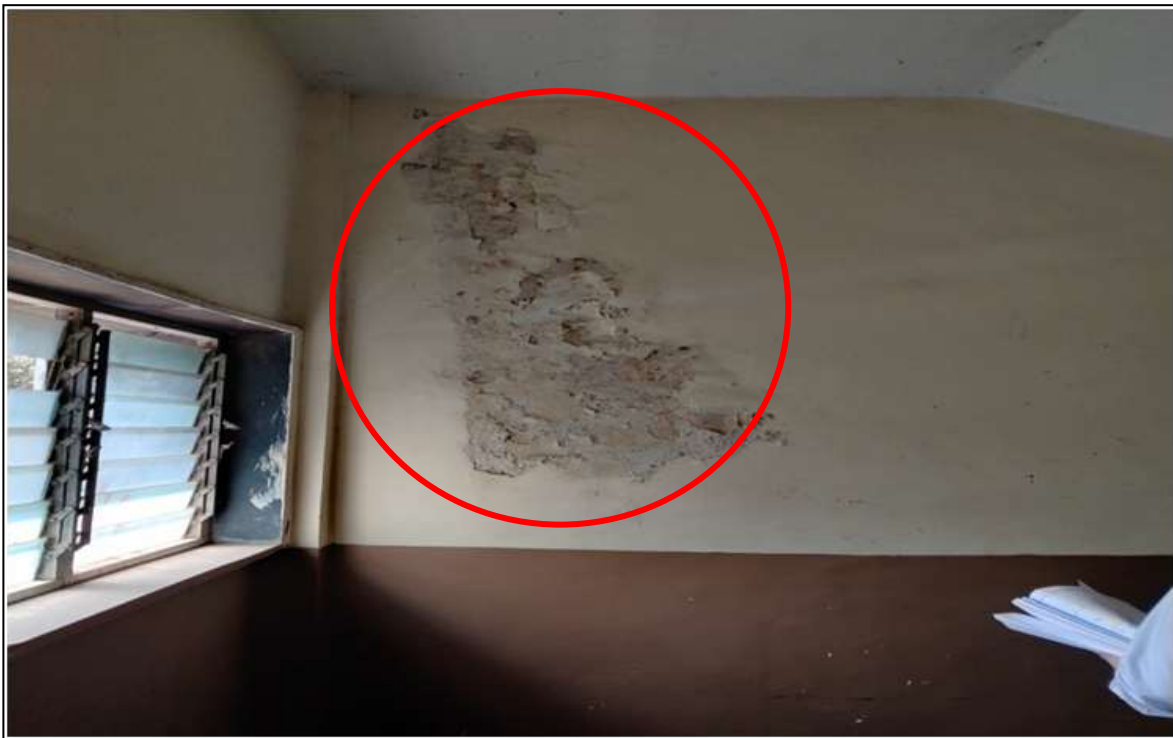
Fig 18. Leakage marks are observed in the staircase area from 2 nd floor to 1 st floor
