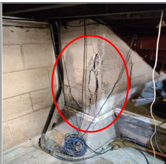
Fig 15. Vertical Deep Crack in column Makeup Room (Ground Floor)
