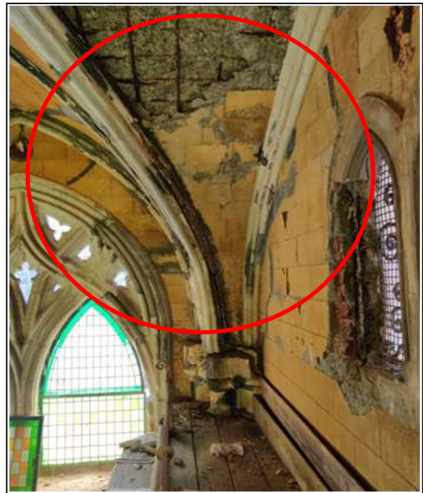
Fig 12. Exposed reinforcement in loft area and falling of concrete.
