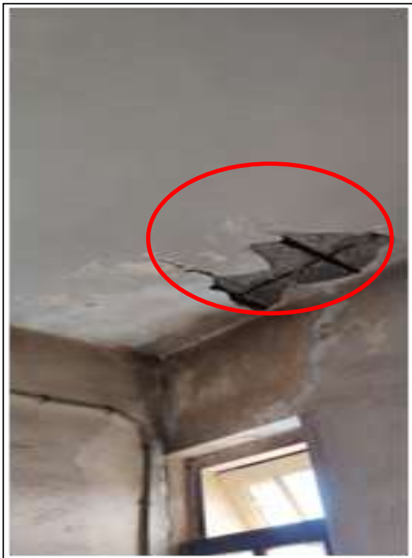
Fig. 26. Lift room exposed slab reinforcement
