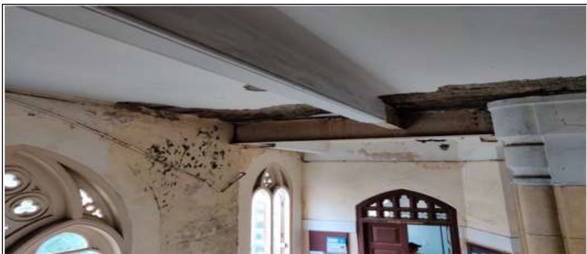
Fig 7. Reinforcement is exposed and plaster is falling in the staircase area between the hall building
