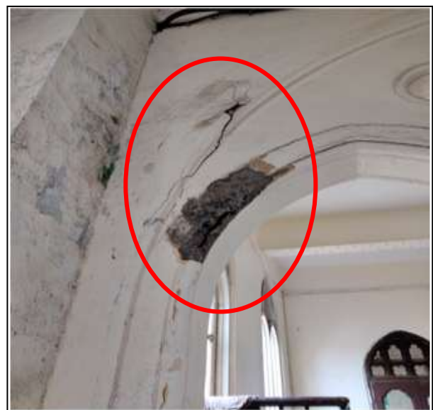
Fig. 16. Exposed reinforcement in the staircase section between Hall Building and Chapel Building at 2nd floor
