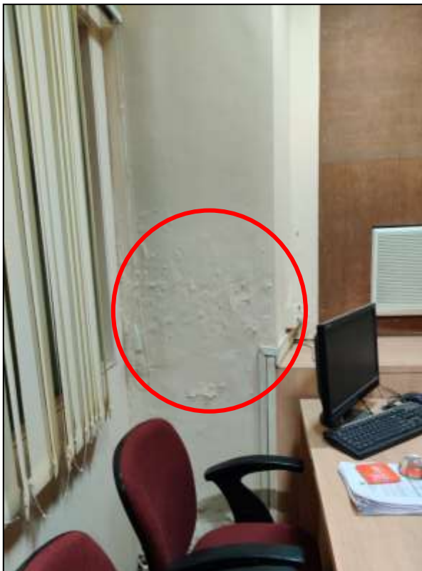
Fig 24. Leakage marks observed in Directors cabin 1 st floor
