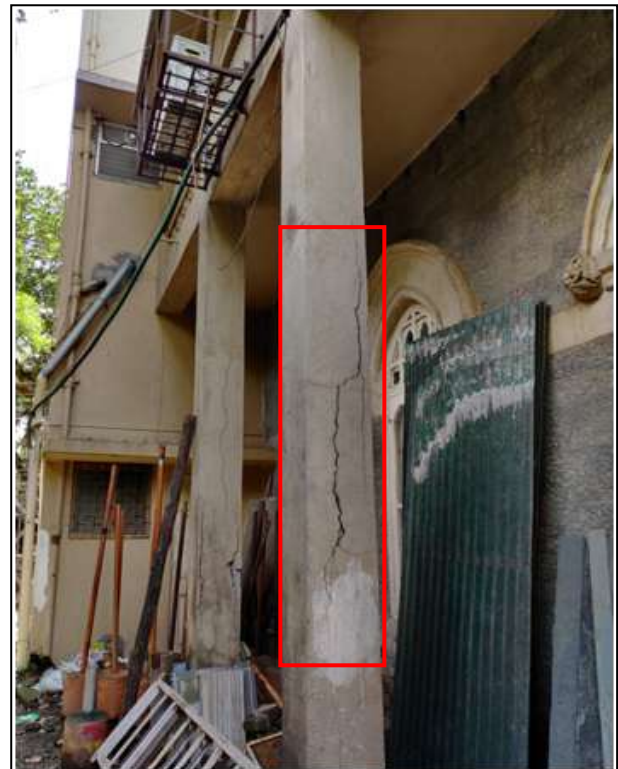
Fig 3. Vertical deep crack in column passage between the admin building and Chapel
