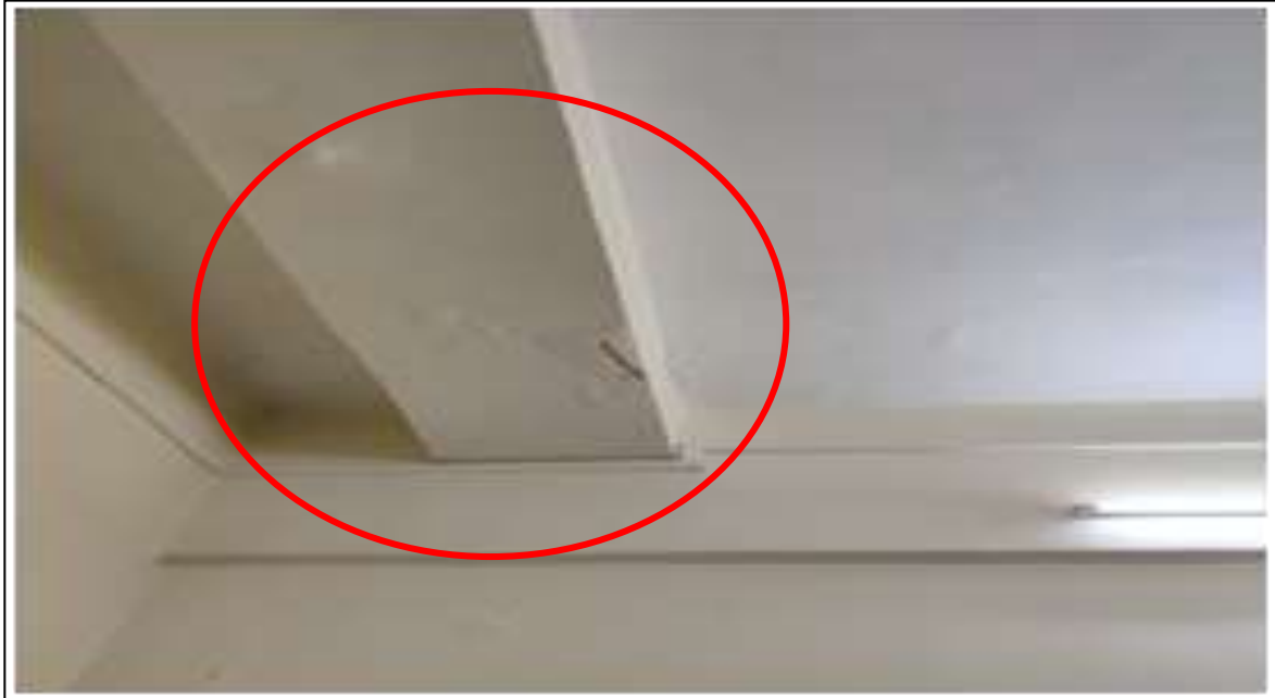
Fig 17. Major leakage in office area 2 nd floor, Gymkhana Building
