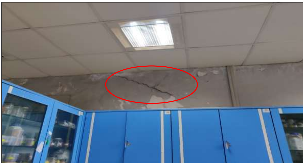
Fig. 8. Deep Crack in the wall of Botany Laboratory 1 external wall (Fourth Floor) Social Science Centre Building
