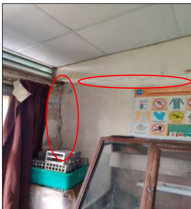
Fig. 9. Vertical and Horizontal deep separation crack in external wall of Botany Laboratory. (Fourth Floor) Social Science Centre Building
