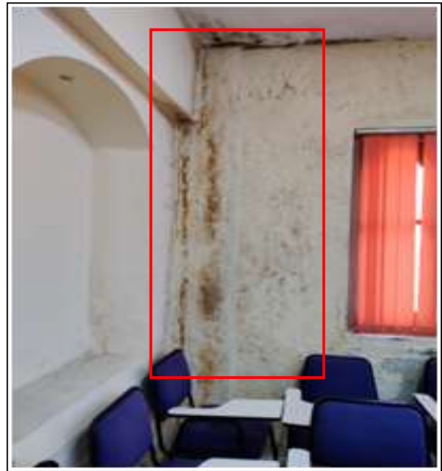
Fig 20. Leakage observed in the wall in the portion near Expansion gap between science building and XIMR building
