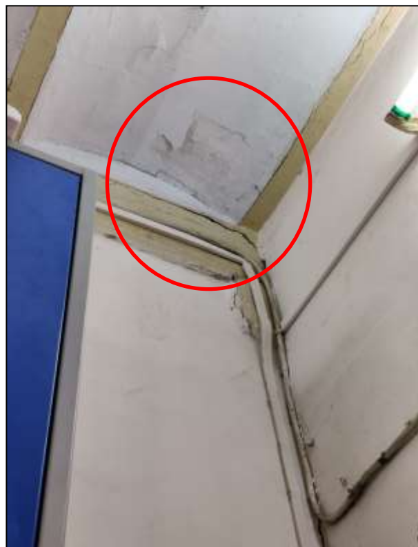
Fig 25. Dampness observed in staircase area
