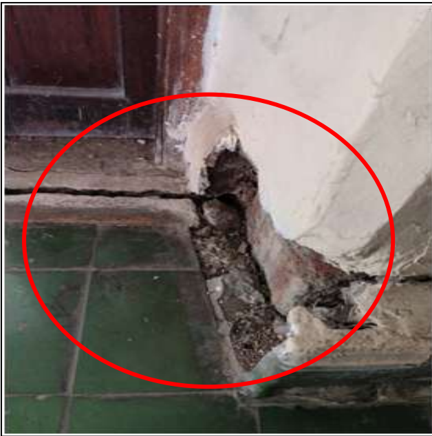
Fig 5. Cracks observed in the floor and wall near the separation crack in hall & science building
