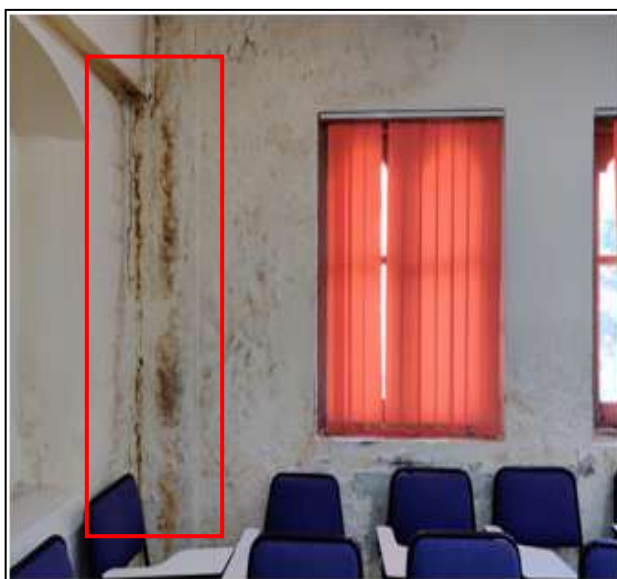
Fig 21. Leakage observed in the wall in the portion near Expansion gap between science building and XIMR building
