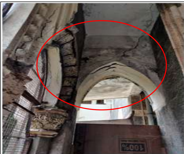
Fig 11. Rusting of Structural Steel Members above vault.
