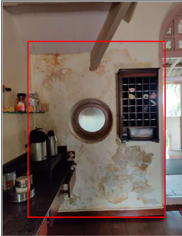
Fig 2. Dampness and leakage marks on third floor Dining room admin building
