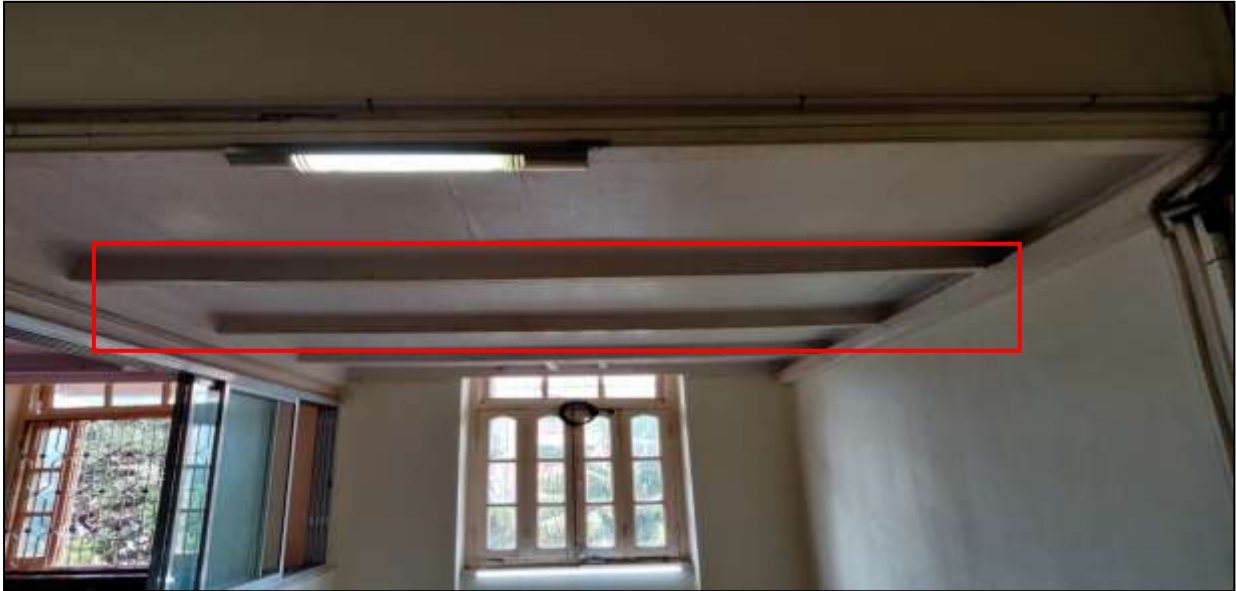
Fig 23. Sagging observed in the wooden beam above staircase area
