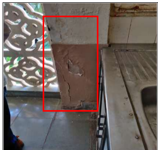
Fig 22. Vertical crack at floor level and Colour peeled off near the expansion joint
