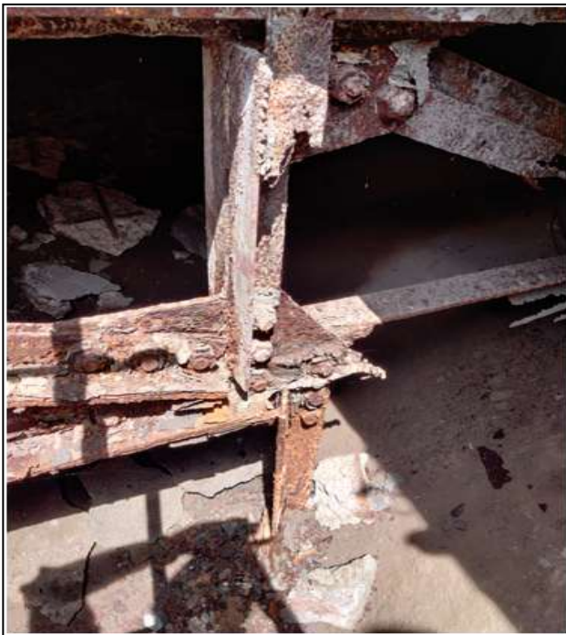
Fig 11. Rusting of Structural Steel Members above vault.
