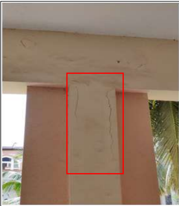
Fig 19. Vertical crack observed in column below the column beam junction 2 nd floor passage area
