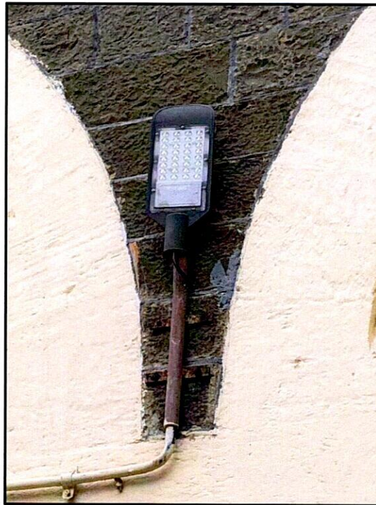
LED Spotlights in the Quadrangle/Basketball Court
