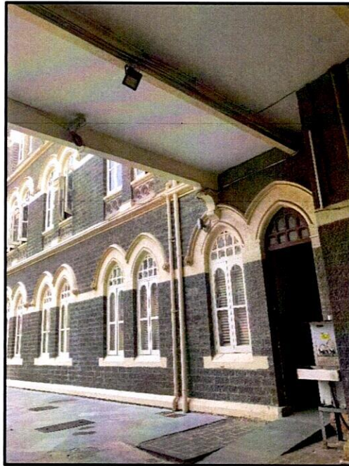
LED Spotlight facing the Side Entrance
