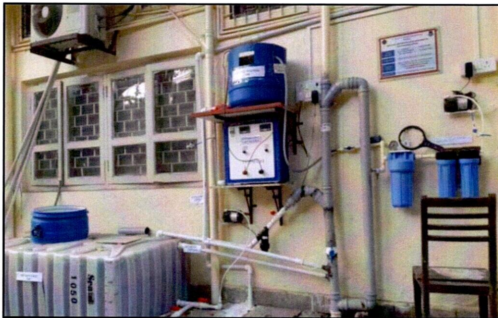
Photograph of the Electrocoagulation Treatment Pilot Plant Site: Back side of Boys' Hostel, St. Xavier's College (Autonomous), Mumbai
