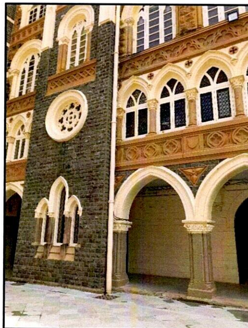
Rainwater harvesting pipe entering ground
