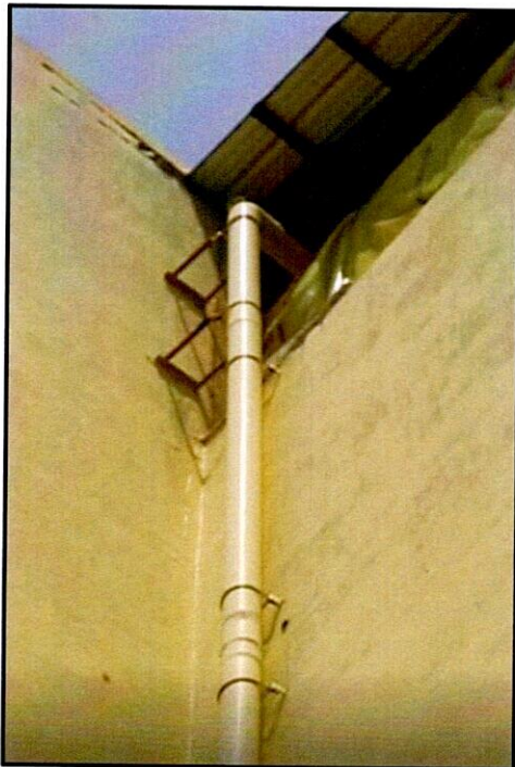
Pipes to carry the harvested rain water to ground level
