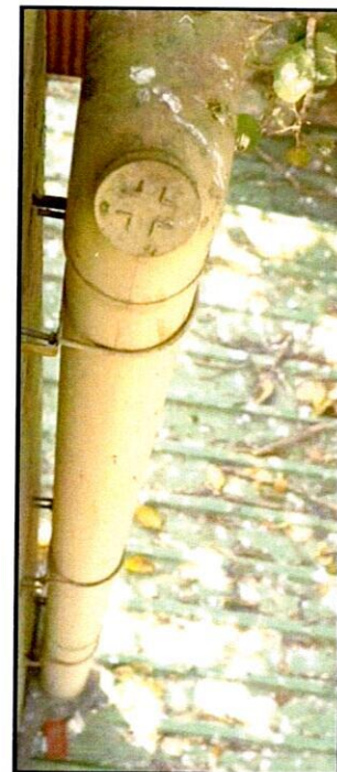
Pipes to carry the harvested rain water to ground level
