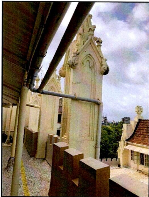
Pipes to carry the harvested rain water to ground level
