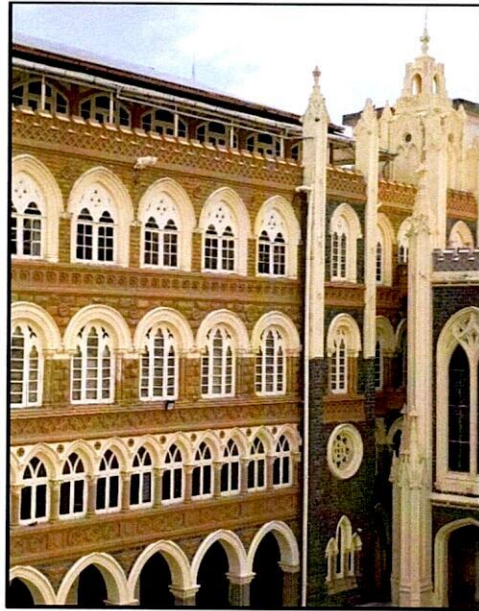
Long shot showing rainwater harvesting pipe reaching ground level from the rooftop
