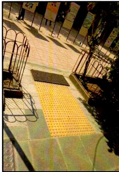
Tactile Guidance Path to help locate exit points and doorways
