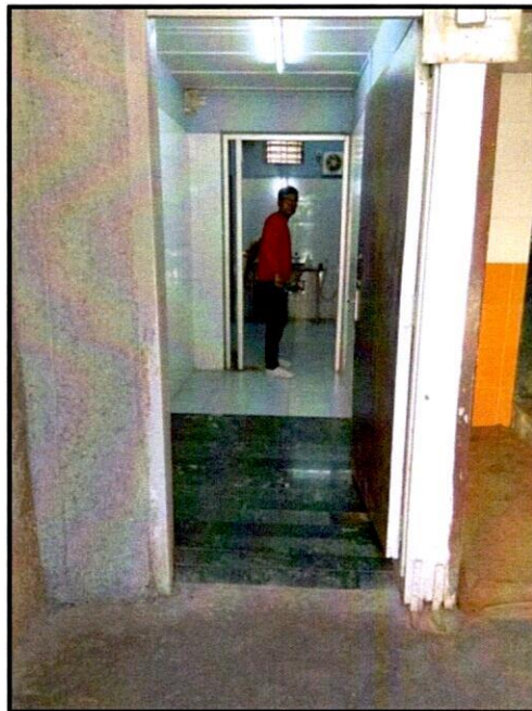
Divyangjan-friendly Washroom Accessible with Ramp
