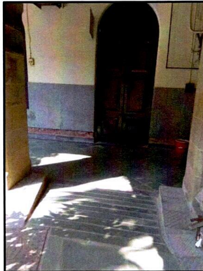
Ramp near the XRCVC.
